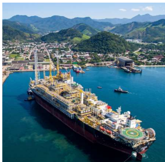
Repsol Sinopec floating platform operating in deepwater Brazil
