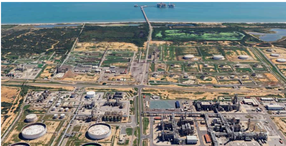
Jose Petrochemical Complex, Anzoátegui, Venezuela (Aerial view)
